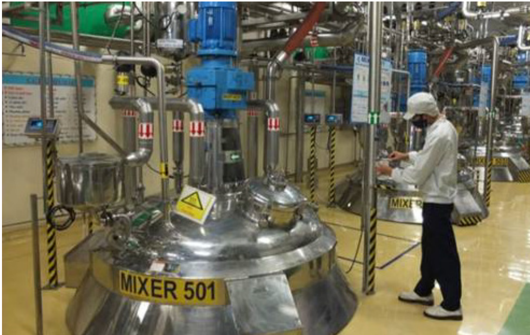
Unilever's factory at Cu Chi near Ho Chi Minh City. Photo: UVN
